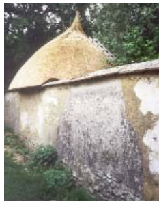
Grade II much repaired witchert wall & attached outbuilding in Haddenham
