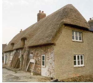
After repairs with new traditional long-straw roof
